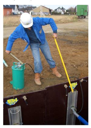
Align the shut frame central to the PERI Fin Ply plate, lower into the trench and swing out.
